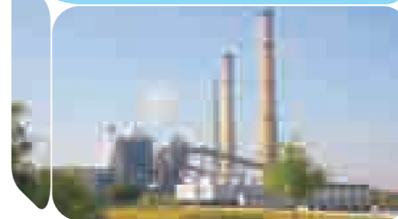
Thermal power plants
